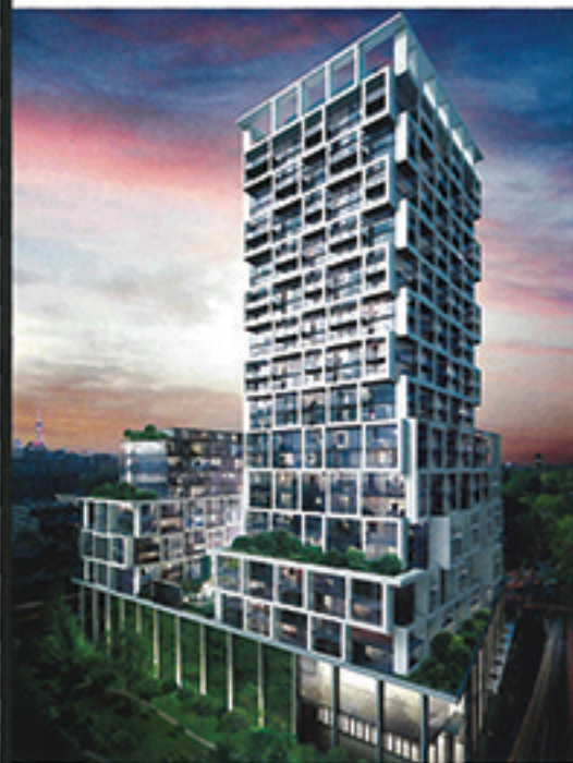
The Art Shoppe is designed by Peter Clewes of architectsAlliance and, with its protruding squares and rectangles, gives the impression of a modern sculpture
